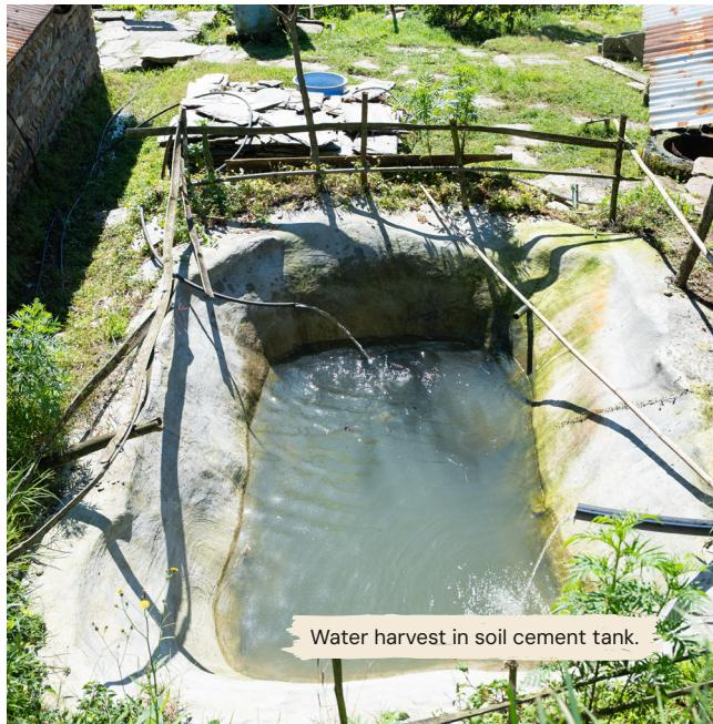
**Water.** Kitchen wastewater is collected in an 800-litre greywater tank, and rainwater in an 8,000-litre soil-cement tank. Both are stored and reused later to irrigate the kitchen garden and vegetables.
