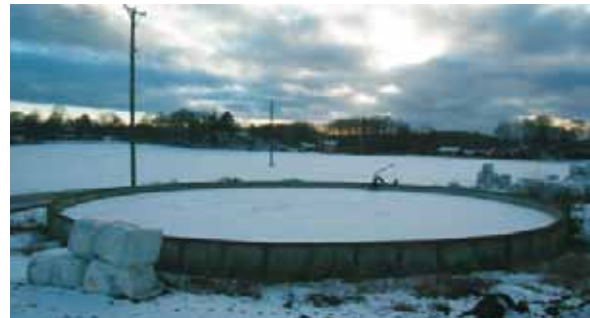
Figure 16: Slurry tank in wintertime, Sweden. This slurry tank will be used for human urine, and it will be equipped with a cover to minimize ammonia losses.
