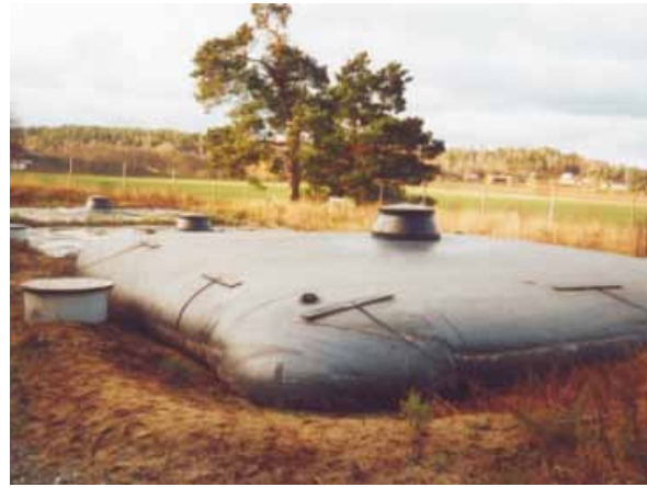
Figure 15: Ready-made large scale storage of urine in Bornsjön, Sweden.
