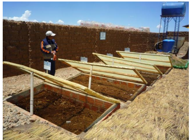
Fig. 6: Composting trenches for treatment of the faecal matter (source: Andersson 2011)
